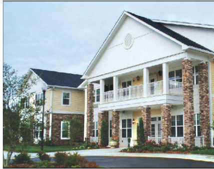
Griffin-American Healthcare REIT III acquired this assisted living property in Mooresville, N.C., along with an assisted living facility in Raleigh in the first quarter, and together the buildings have 124 units. The properties were part of a five-building portfolio, and the REIT expects to acquire the remaining three in the coming months.
